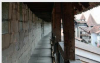
The rampart walls were built in several stages and from a variety of materials such as gravel, tuff and sandstone. The lower 15 layers of stone date from before the town's construction (12th century).
